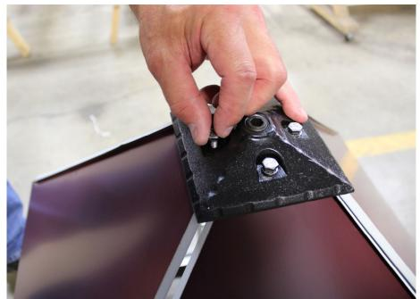
Using gloves, slide the corner connectors on each corner of the roofline as shown. Use putty knife to guide Connector under Roof Cap. (See Picture 13.)
