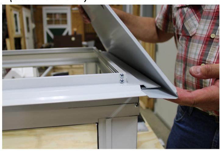
Continue with the next two roof panels as in *Step #9*. Align the bottom 45 degree cut toward the outside at the roof panel corners. (See Picture 9.) Leave the 4<sup>th</sup> panel off for now.
