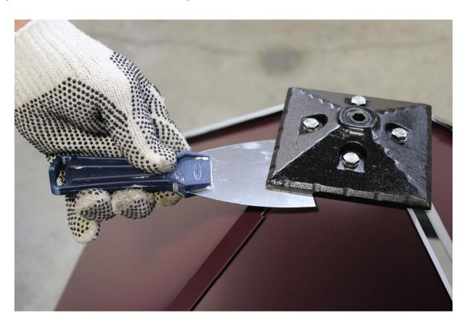
The tail end of the connectors extend past the corner of the roof unit approx. 1".
