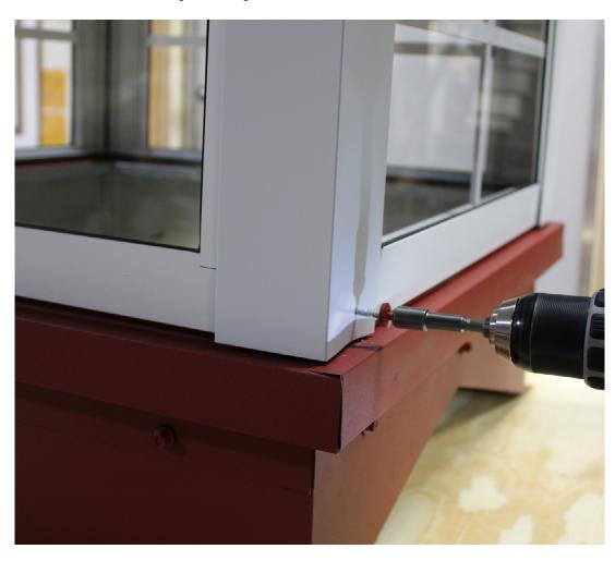
To fasten roof unit to sides unit, install #10 x 1" white self-drillers with washers in prepunched holes between roof and lited side on all four sides.
