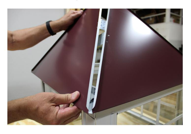
Start the Roof Cap attachment by aligning it with the top of the Roof Panels and inserting cap bolt through the Roof Cap and the panel holes then thread into the Cap Base. Leave the cap bolts loose so the last panel can be inserted. (See Picture 10.)
