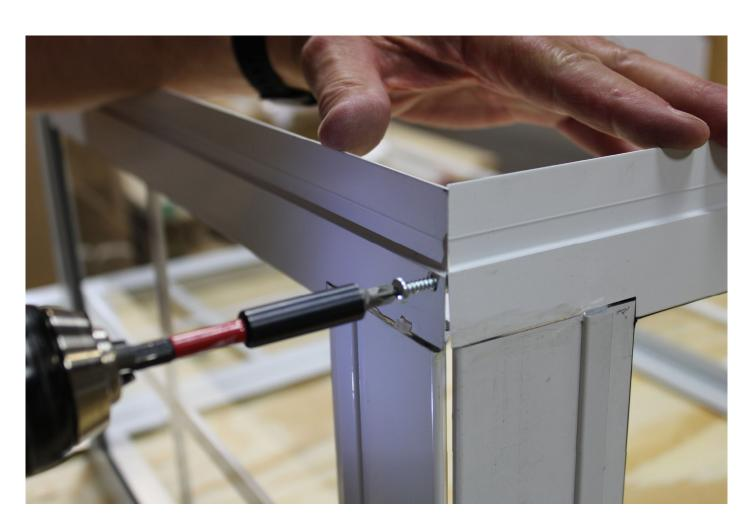
Using the #8 x 1" PPH (Philips Pan Head) screws provided, drive the screws through the hole at the edge of one Side Panel into the screw bosses (i.e. the small channels) of the second Side Panel to form a 90-degree angle.
