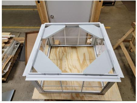
Mount side assembly on curb base with screws. If custom curb base is built see *Cupola Box Guidelines* for proper dimensions.
