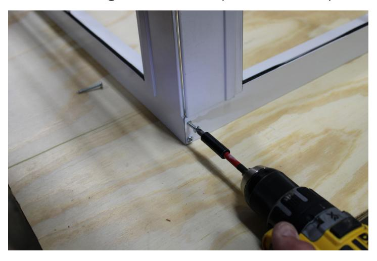
Place the 3<sup>rd</sup> Side Panel at the edge of the 2<sup>nd</sup> Side Panel and attach in the same method as before. (See Picture 3.)
