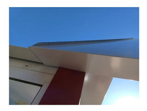
Make sure the Roof Panel top tab is between the Roof Cap and the Cap Base and holes are aligned properly under the Roof Cap. Apply the last cap bolt to the roof cap. Do not tighten at this time. (See Picture 12.)
