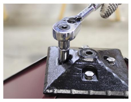
Install eight (8) #12-14 x 1" hex head self-drilling screws ¾" from lited side panel and 3 ½" to 4" from each roof panel corner, and upward into internal roof framing to add rigidity to roof assembly.
